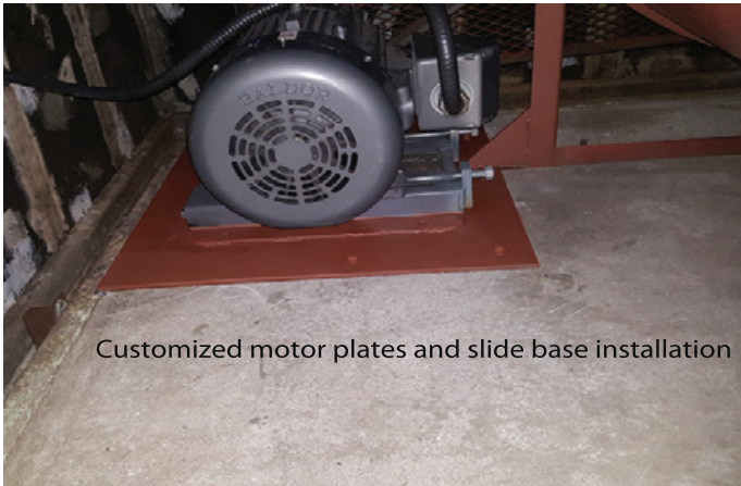
Fluxdrive Magnetic ASD Conversions on 16 Exhibition Hall Fans
