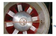
**Solution to Fig. 3** Installed Brand New Controllable Pitch Fan & Repaired Motor.
