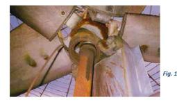
**Solution to Fig. 1** Replaced both Fan Bearings & New Motor Required.
