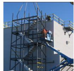
Ladders, Platforms, Handrails, & Doors
