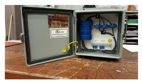
Figure 3 = 10 HP VFD/Junction Box - AHU
